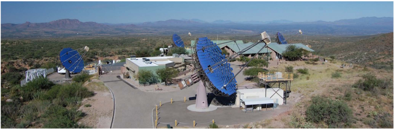
Figure 1. Elevated view of the VERITAS array located at the base of Mount Hopkins near Tucson, AZ. Pictured are the four individual telescopes, which are roughly 100 m apart, the Fred Lawrence Whipple Observatory visitor center, and the VERITAS control building (with the white roof). Image from Abeysekera et al. (2016).
