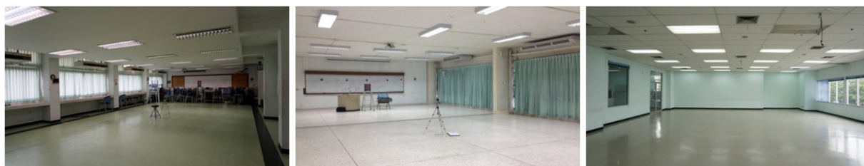
Figure 4. Display floor, walls, and ceiling materials of the large classrooms in KMITL
