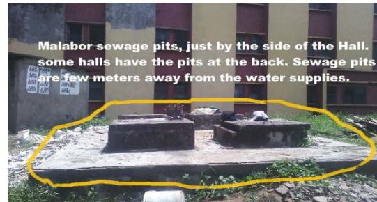
Photo 2. Sewage pit for one of the halls in Malabor hostel
