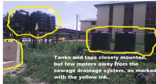
Photo 1. Mounted tanks and taps in Malabor hostel halls
